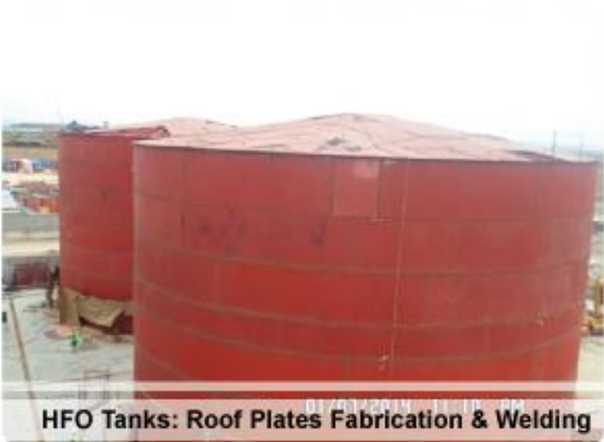
Fabrication & Erection of Tank Roof Structure
